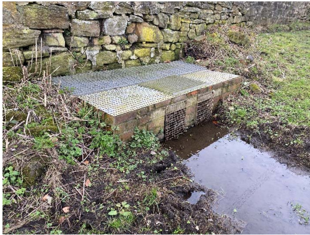
Photo 1: Culvert under Lamesley Road (TN2)
